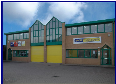
Bracknell, Berkshire Head Quarters
